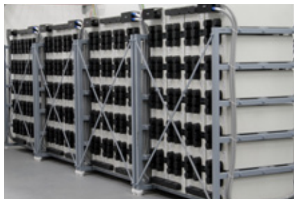
Energy Storage System
